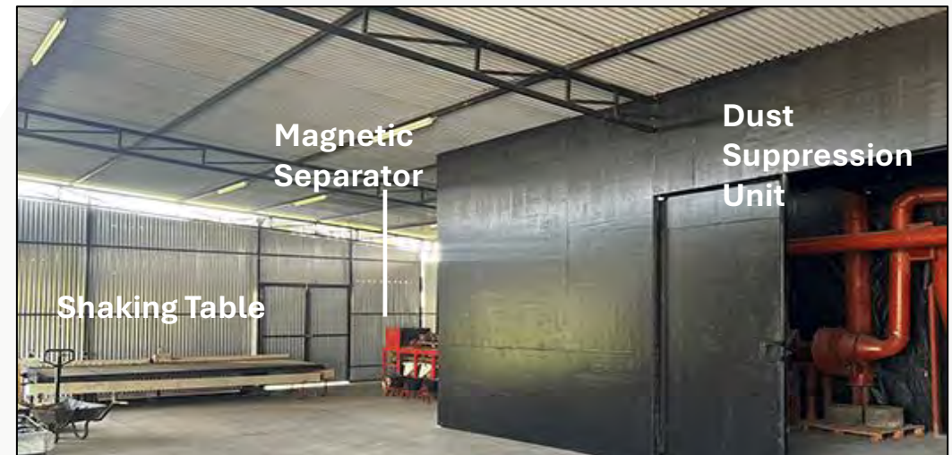
Aterian Upgrade Facility (Comptoir) in Kigali
